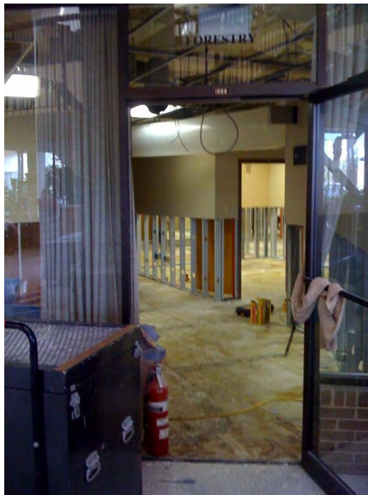
Figure 27: Office of Forestry after Hurricane Gustav
